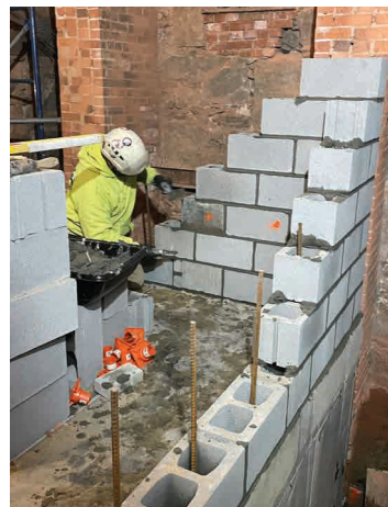
▲ Building the elevator shaft.
