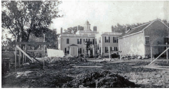
▲ Construction on the Mayflower Society House in the 1930s.
