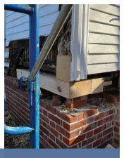
"Foundation corners throughout the House had settled and shifted requiring the rebuilding of stone and brick support walls."
